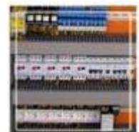
Electrical components from well-known European
